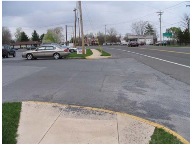
Example of a driveway entrance that functions like an intersection (in the Town of Stephens City). In this example, it is recommended that crosswalk markings be added. The detectable warnings do not meet the requirements of the Americans with Disabilities Act Accessibility Guidelines.
