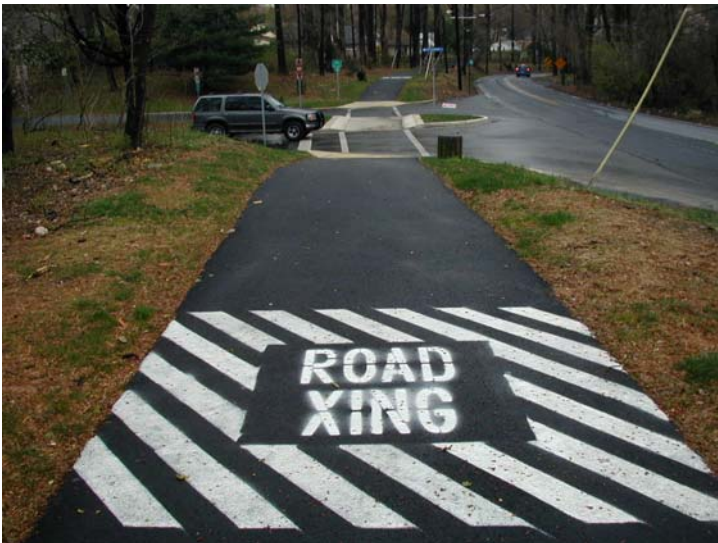
Example of an intersection treatment on a sidepath
