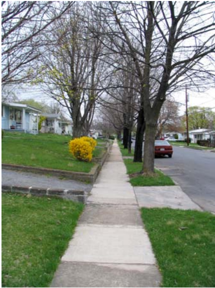
Example of a sidewalk continuing over a driveway in Winchester, VA.
