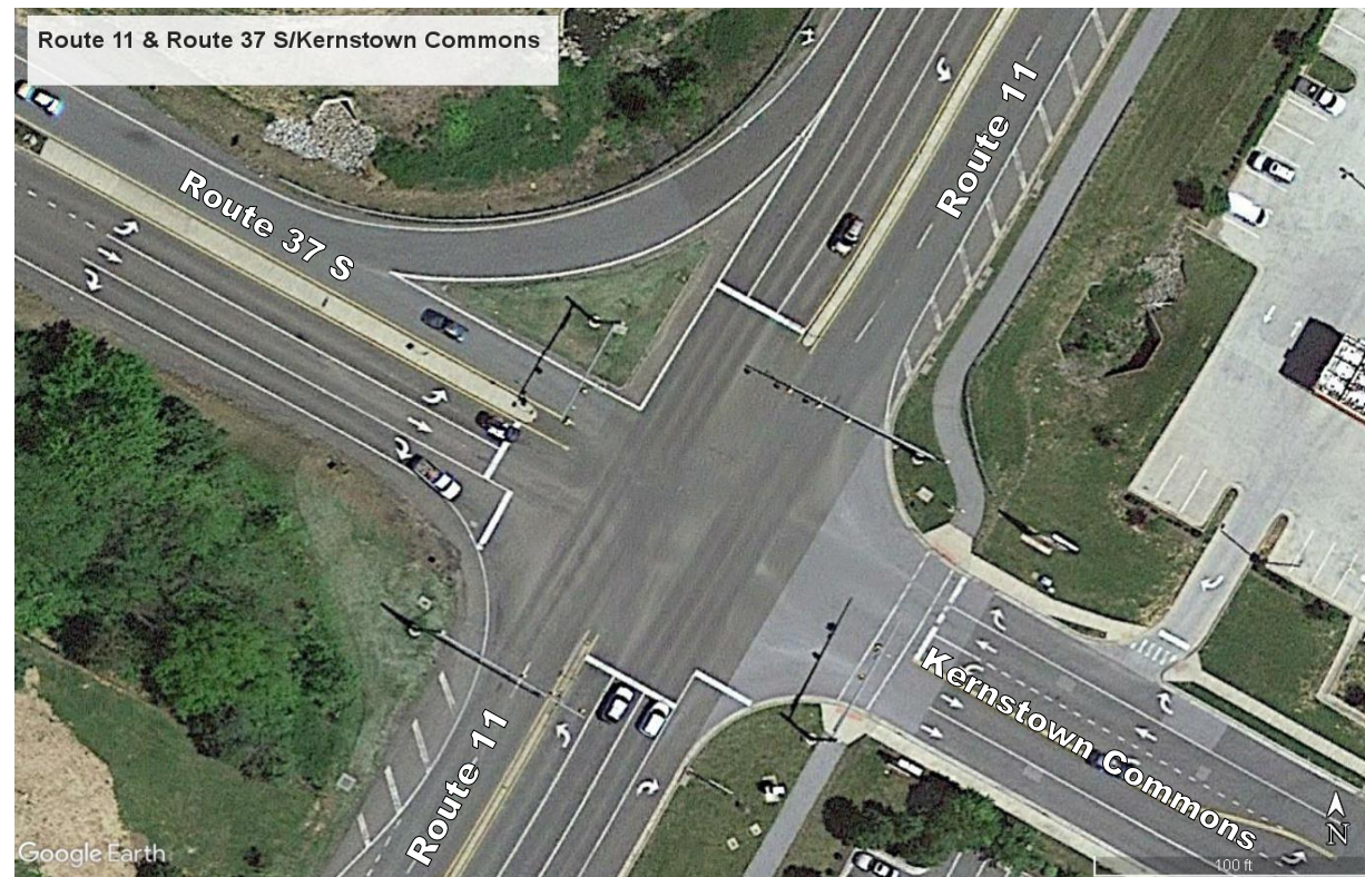
Figure 11: Route 11 at Route 37 S (EB) On and Off Ramp / Kernstown Commons Blvd
